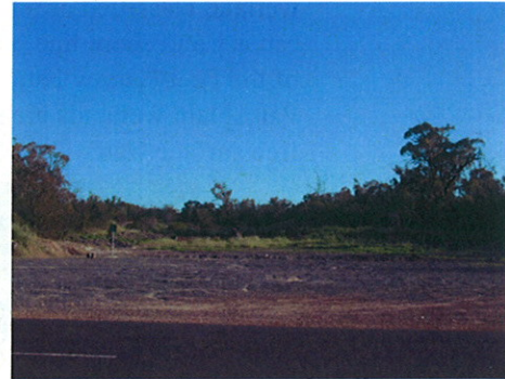
Photo 5. Cleared compacted area
