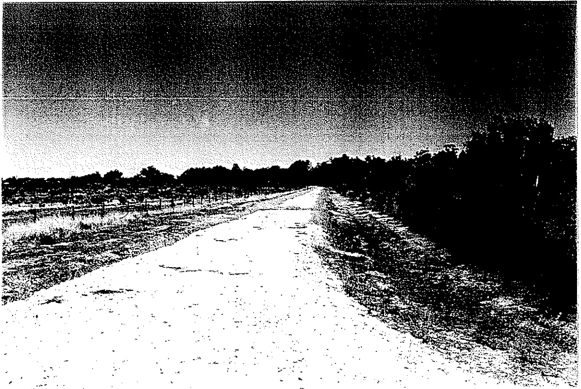
Plate 1: Newly constructed access drive that can be used for road access. Facilitated by land swap with Location 2986.
