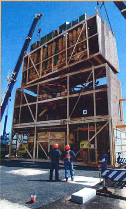
One of Iluka's concentrators being reassembled following relocation
