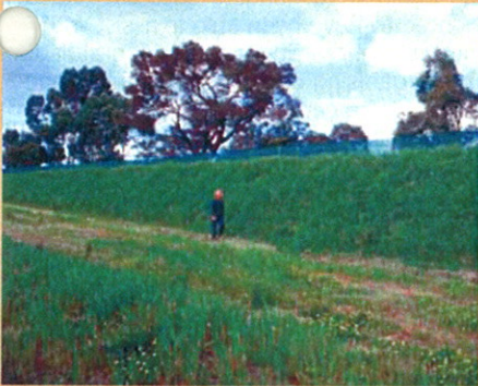
An example of a topsoil bund wall
